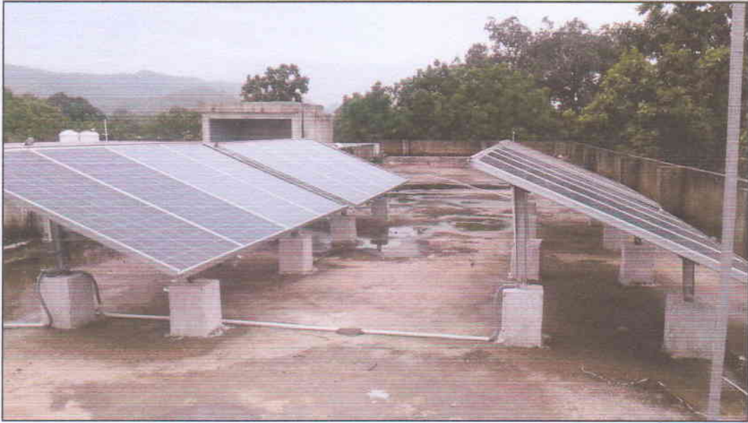
Figure - Solar PV at roof of facility
