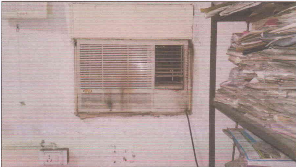
Figure - Window AC installed in facility
