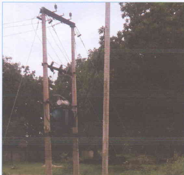
Figure – Transformer installed in facility
