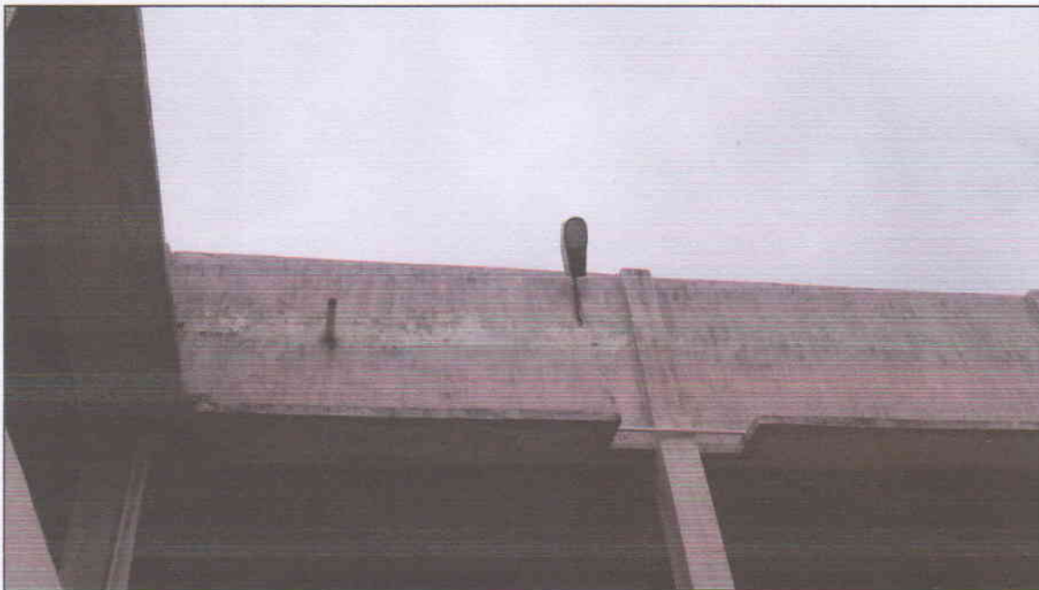
Figure - Exterior light installed in facility
