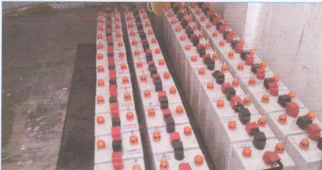
Figure - Shows battery installed in facility
