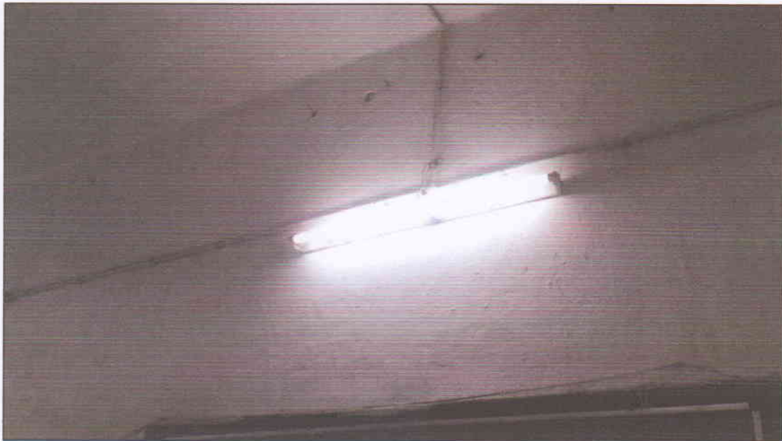
Figure - Fluorescent tubes installed in facility
