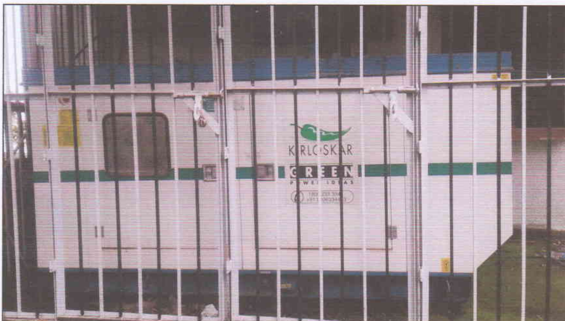
Figure - DG installed in facility
