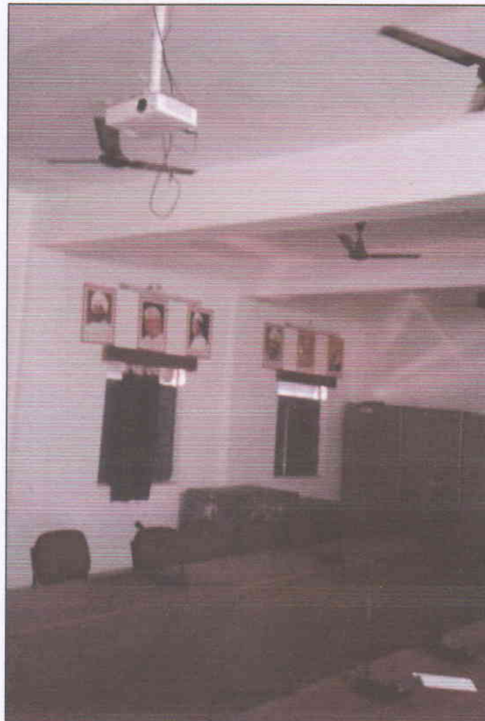
Figure - Projector & Mic System installed in facility
