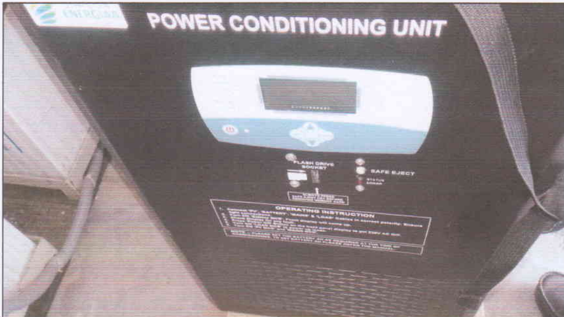
Figure - Solar PV meter in facility
