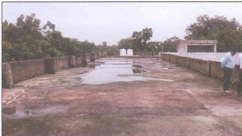
Figure - Roof of facility
