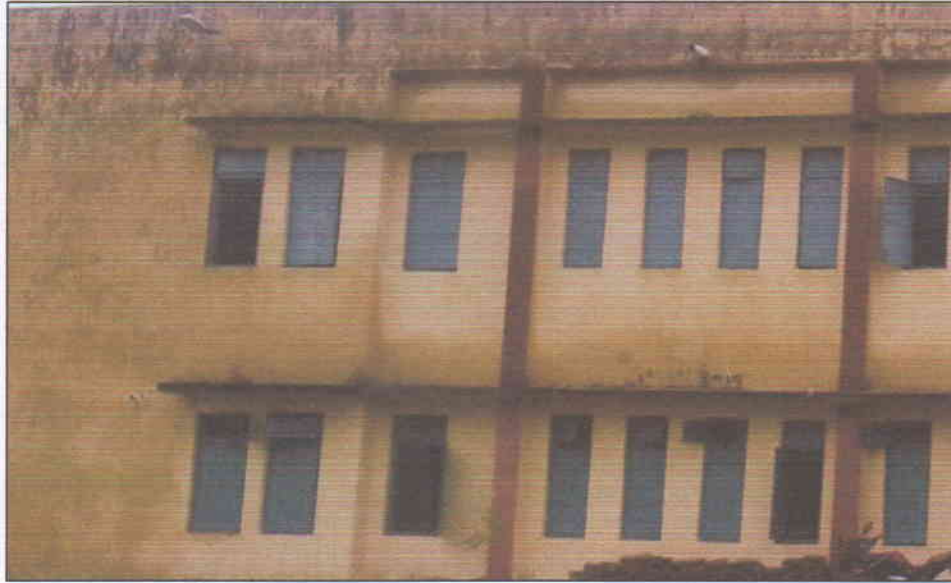
Figure - Shows Wall of Facility
